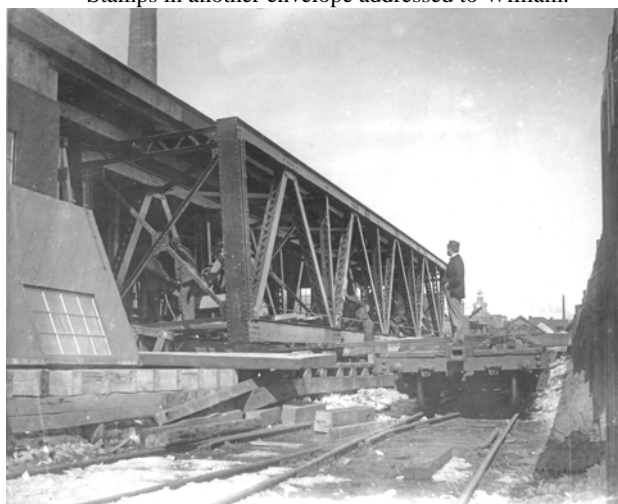
William Law directs the loading of a sixty foot double truss on to a CPR flat car at the Dalhousie Street bridge works. (Ivan Bateman)
