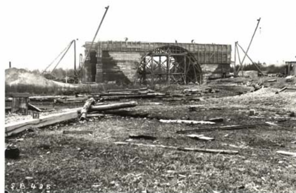
Arched reinforcing rods for the bridge – TSW Archives Progress on the Canal Lake arch bridge
