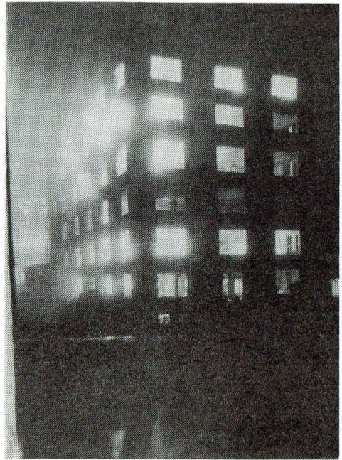
The burned out shell of the "fire proof" warehouse.
